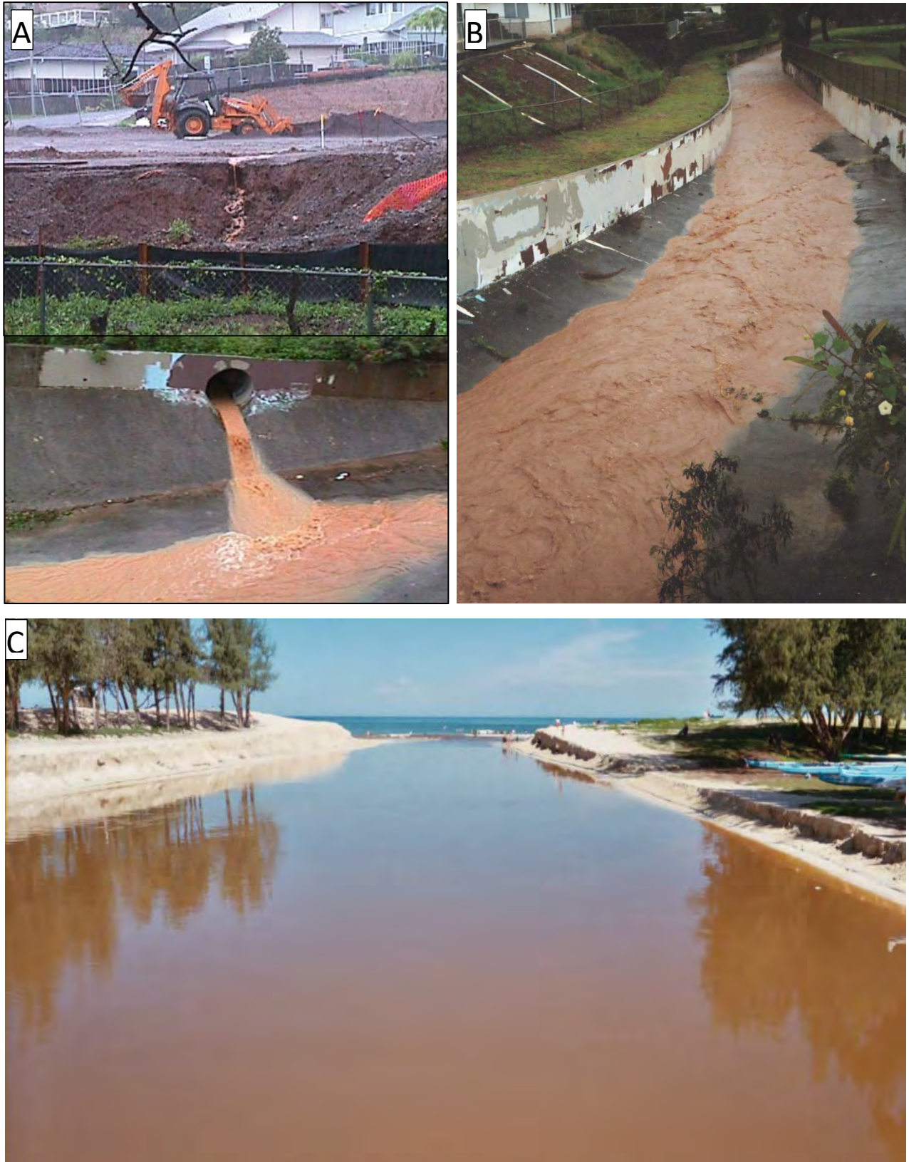
Figure 20 Construction activities (A) have the greatest impact upon delivery of sediment and nutrient turbidity to the pond (B) and into the ocean (C) when the stream mouth is open.
