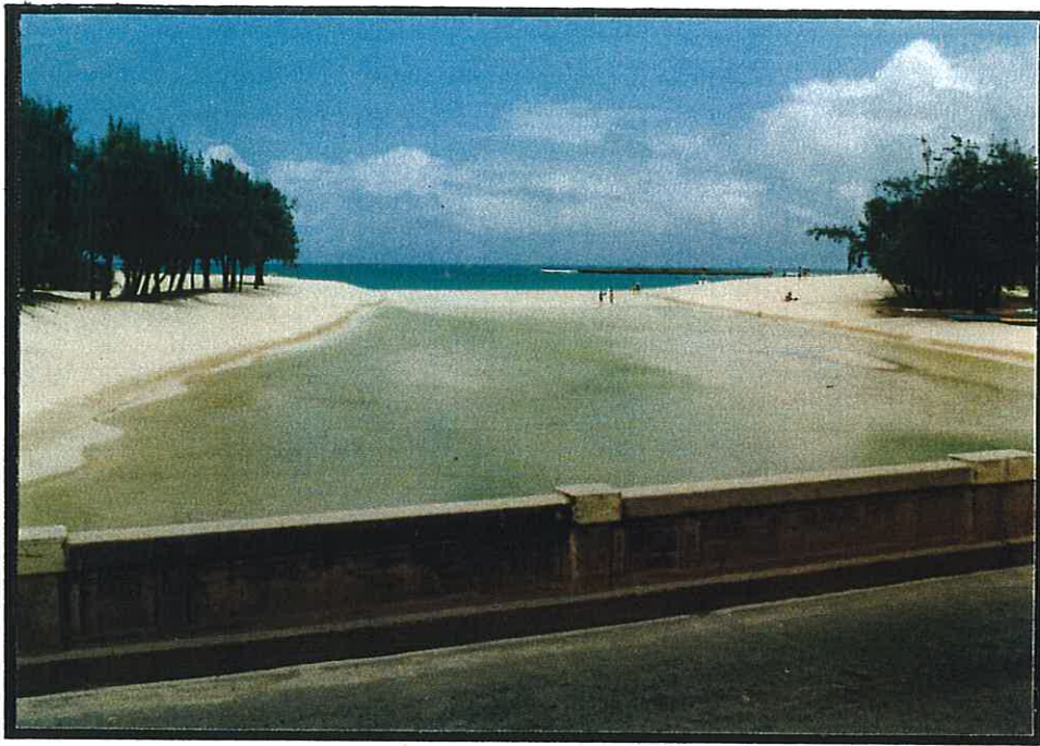
Photograph No. 1 : Sand Berm at Kailua Beach
