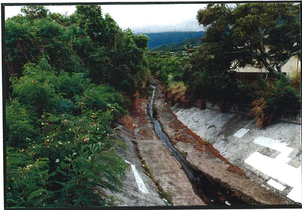
Photograph No. 5 : Ditch Connecting Kaopa Basin to Enchanted Lake
