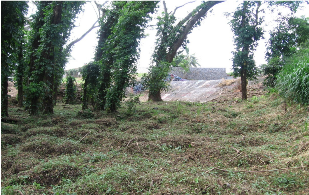
Photo 1-49 Apparent spillway from Kapaa Silt Basin toward City debris control structure.
