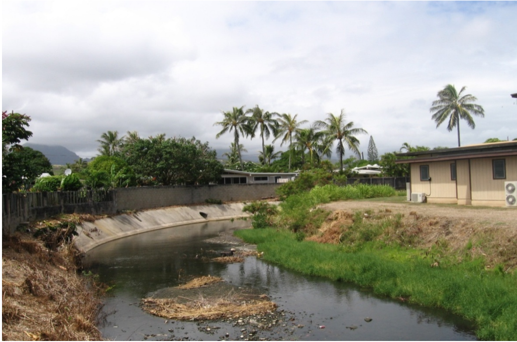
Photo 1-26 Hele Drainage Channel looking downstream. Note large Mango Tree, Alahaki Street outlet, sediment deposits with vegetation growing on the north bank, gross debris within channel, and dead grass (sprayed) on south bank.
