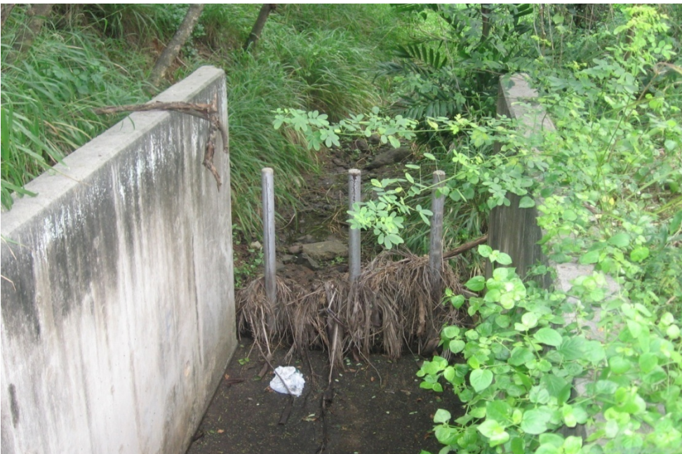
Photo 1-12 Intermittent stream from Kailua High Schools general area ends and Akipola Lined Channel begins at vegetation barscreen BMP.
