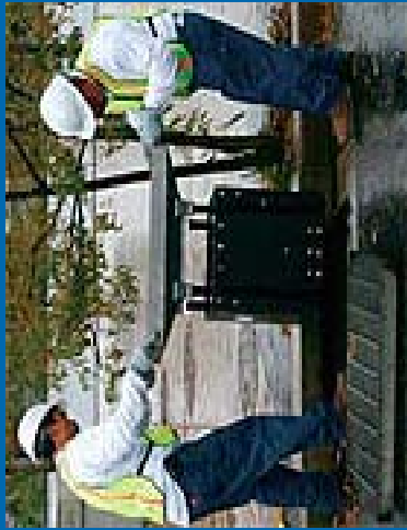
Installation of the Ultra-Urban Filter with Smart Sponge®.
