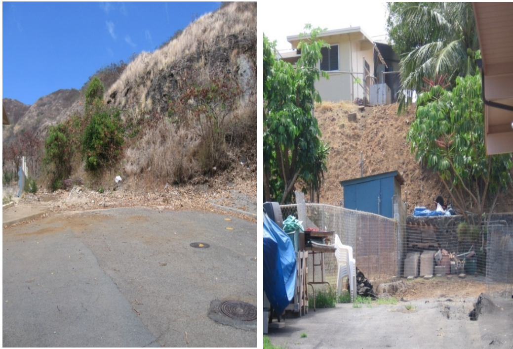
Photo 1-32 and 1-33 Road debris and barren slopes along Kupau Street in the southeast corner of the WKIP 10 drainage area were common observations for this drainage area and the others in this study.
