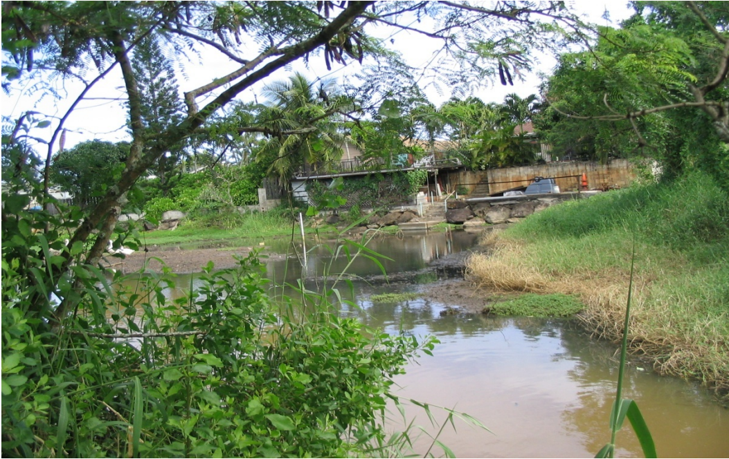
Photo 1-39 Approximate location of WKIP 44 outlet; sediment buildup in this area continues to alter the outlet location.
