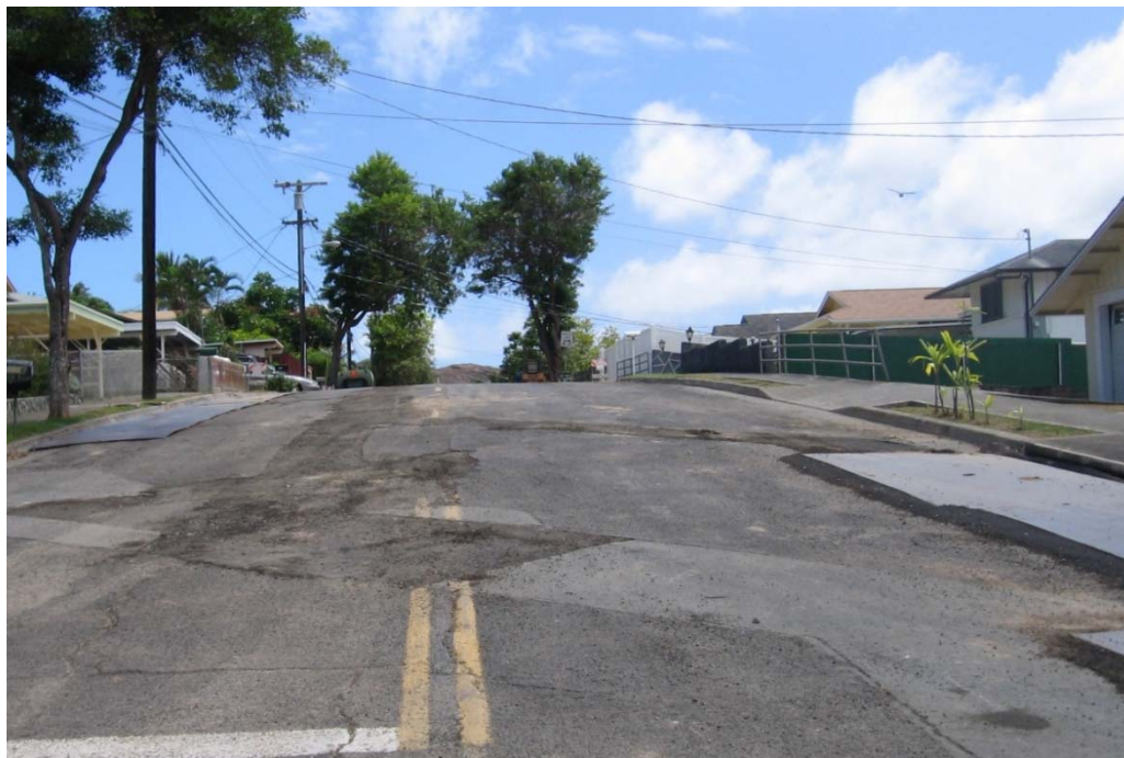
Photo 1-34 Road construction on Loho Street looking southeast.
