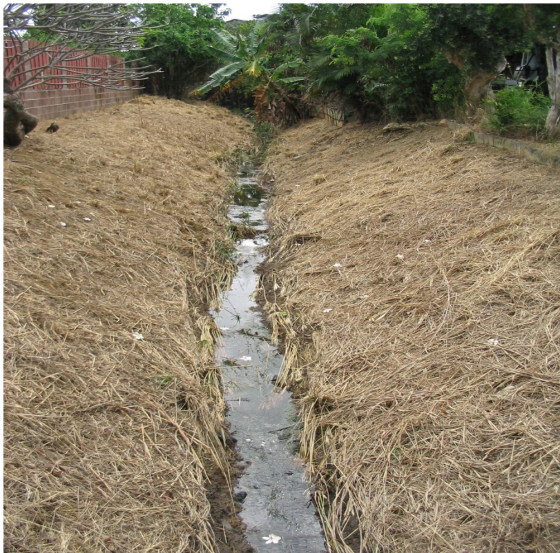
Photo 1-5 Photo from Kahili Street Bridge looking south at bend up Alahaki Ditch. Note lined embankment and excessive growth.
