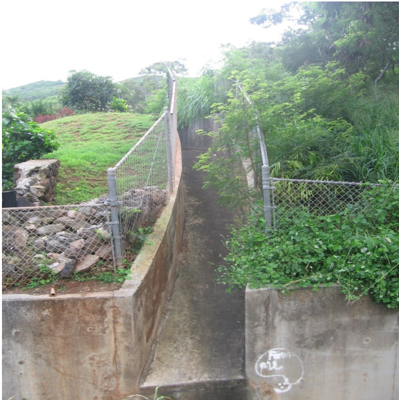
Photo 1-11 36-inch concrete ditch intersecting upstream portion of Akipola Lined Channel.
