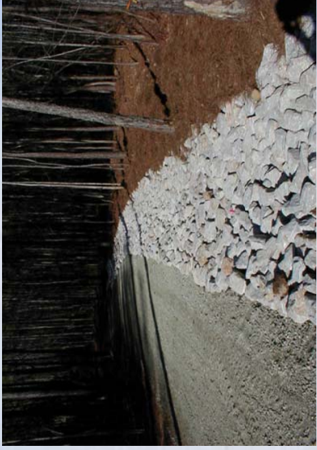
Riprap can be used to filter stormwater from residential, commercial or runoff areas.
