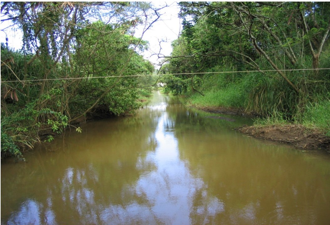
Photo 1-40 Unlined portion of Keolu Drainage Channel.
