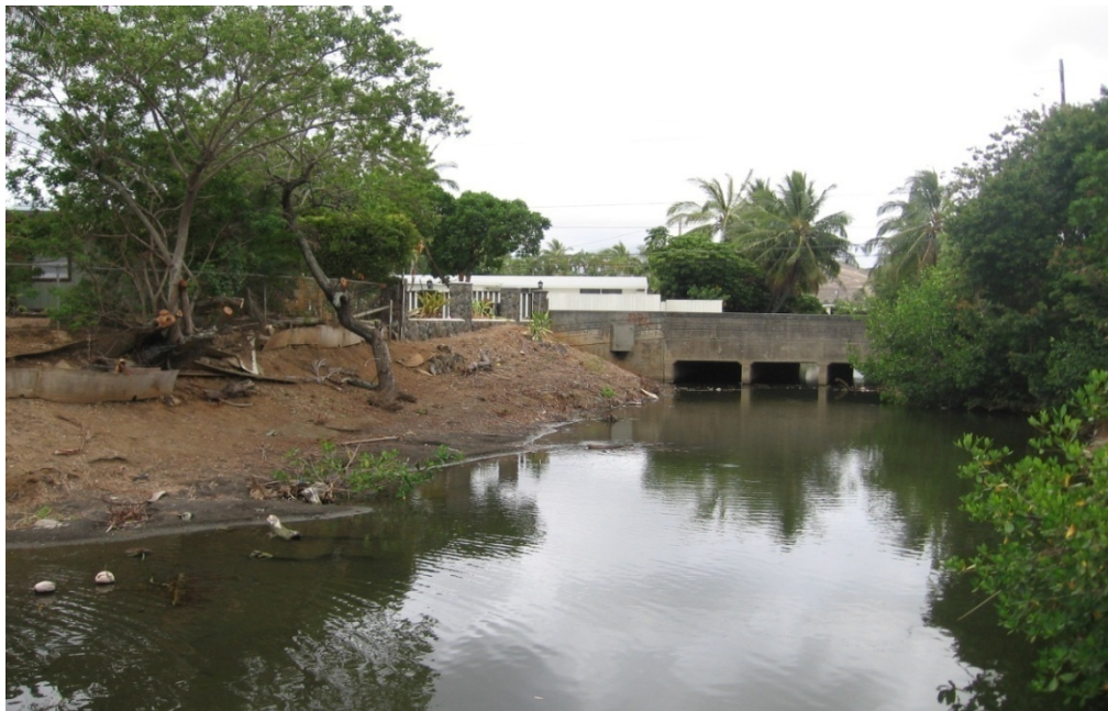
Photo 1-18 WKIP 10, Hele Channel looking north at Akumu Street Bridge from Kamahele Ditch junction. Note sediment build up and barren embankment. Recommended bank stabilization area using vegetative riprap and/or mechanical revetment .
