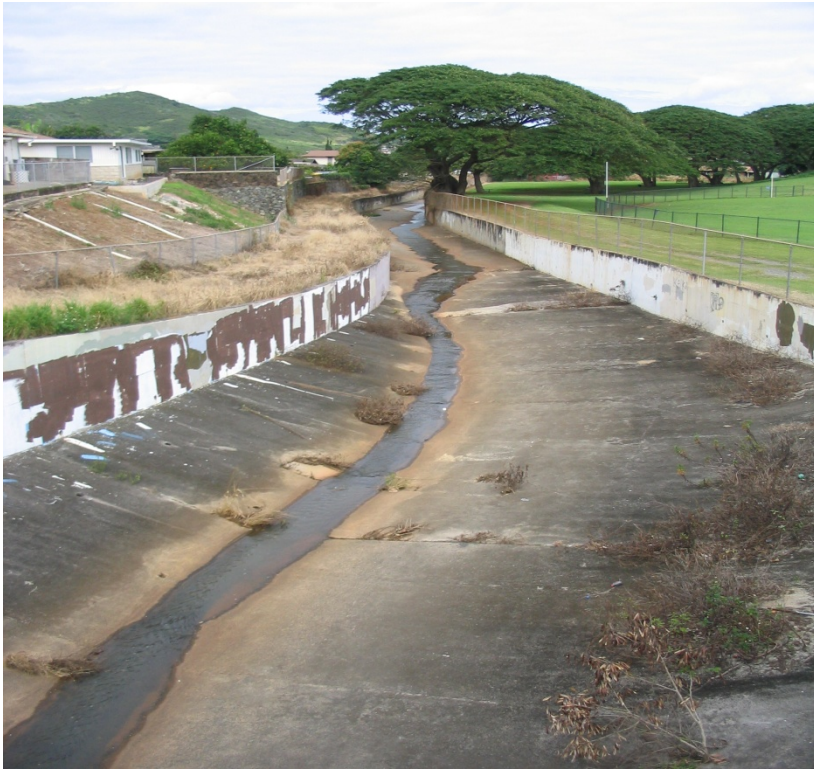
Photo 1-43 Keolu Lined Channel looking downstream (north) from Keolu Drive.
