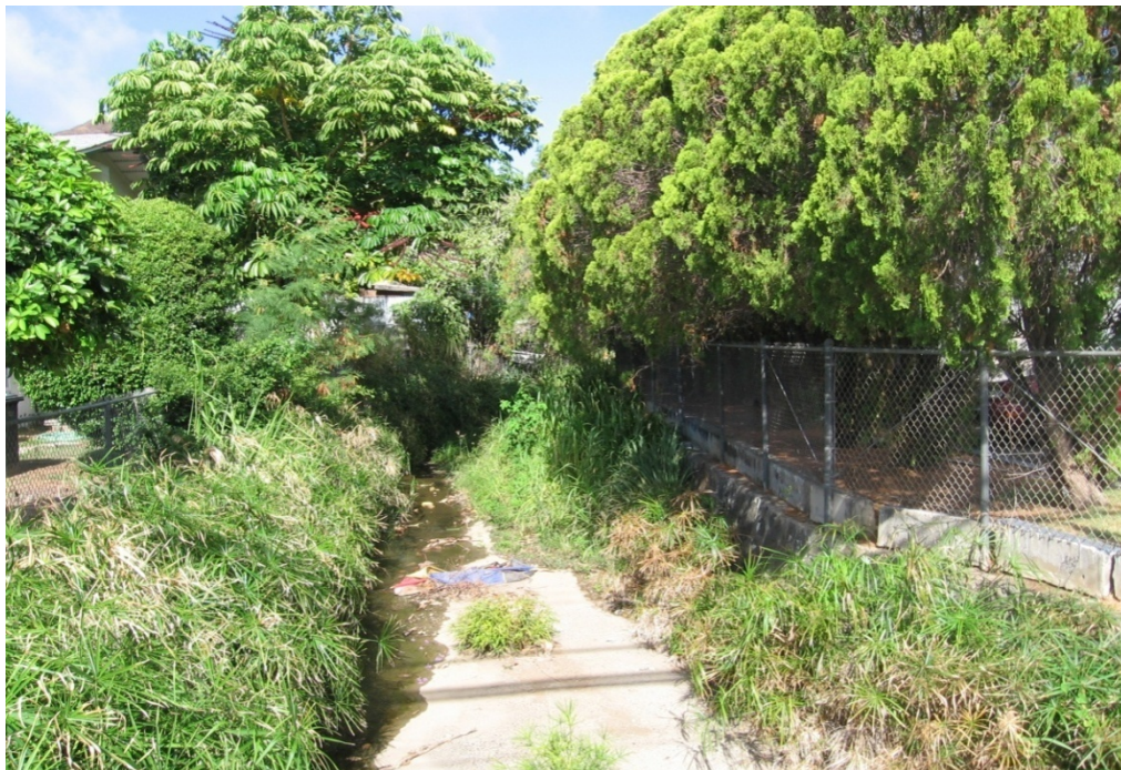
Photo 1-29 Hele Drainage Channel looking east from Keolu Drive. Tenn's Auto is the property adjacent to the south.
