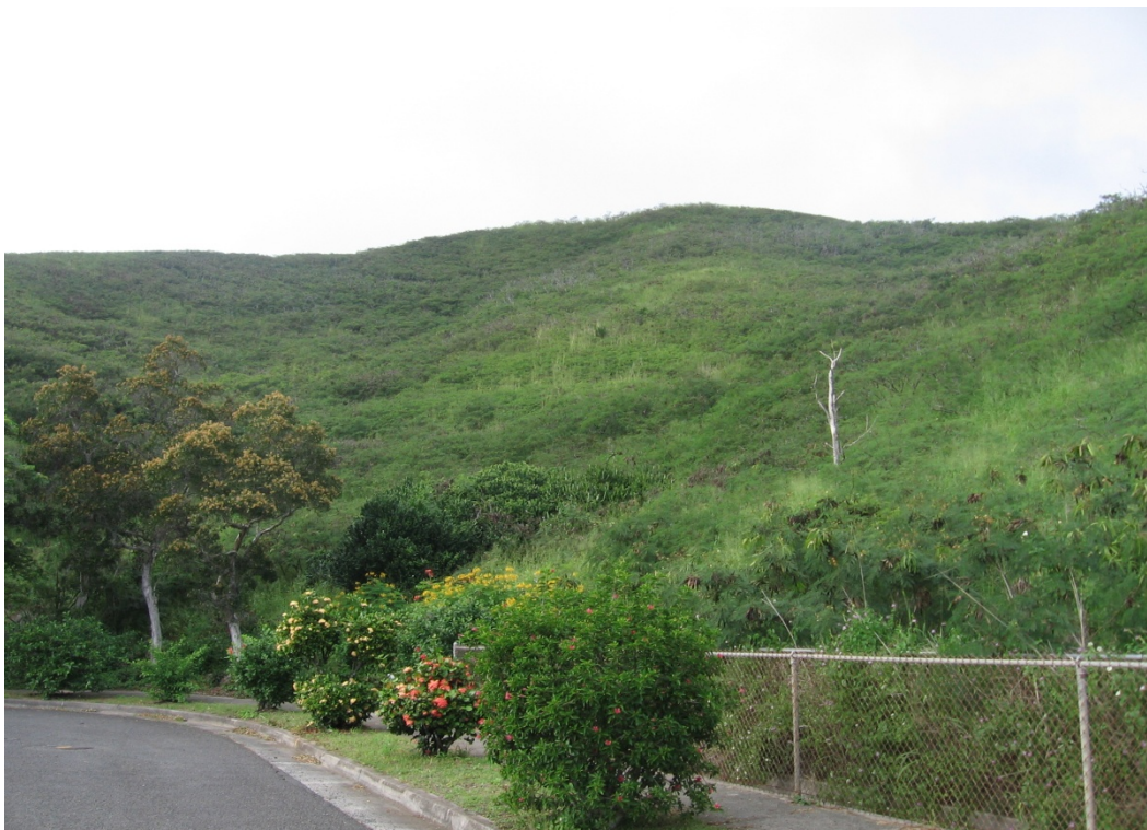
Photo 1-13 Typical vegetative hill “source area” associated with WKIP 52 drainage area. A 24-inch concrete ditch runs parallel to fence and Akiohala Pl. (Photo 1-15).
