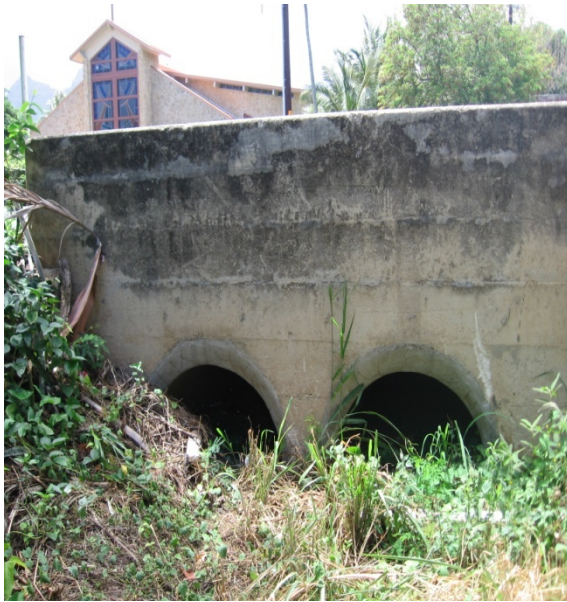
Photo 1-23 Kamahale Ditch looking southwest toward Keolu Drive pipe culvert.
