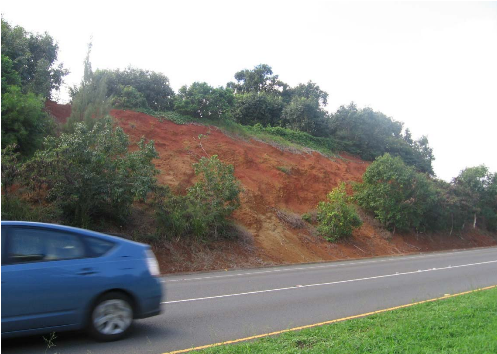
Photo 2-3 Steep, barren embankments along K-Hwy are common.
