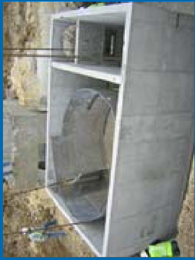
The Vortechs Stormwater treatment system.
