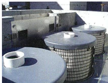
A shallow concrete vault configuration of three FloGard® PERK FILTER cartridges.
