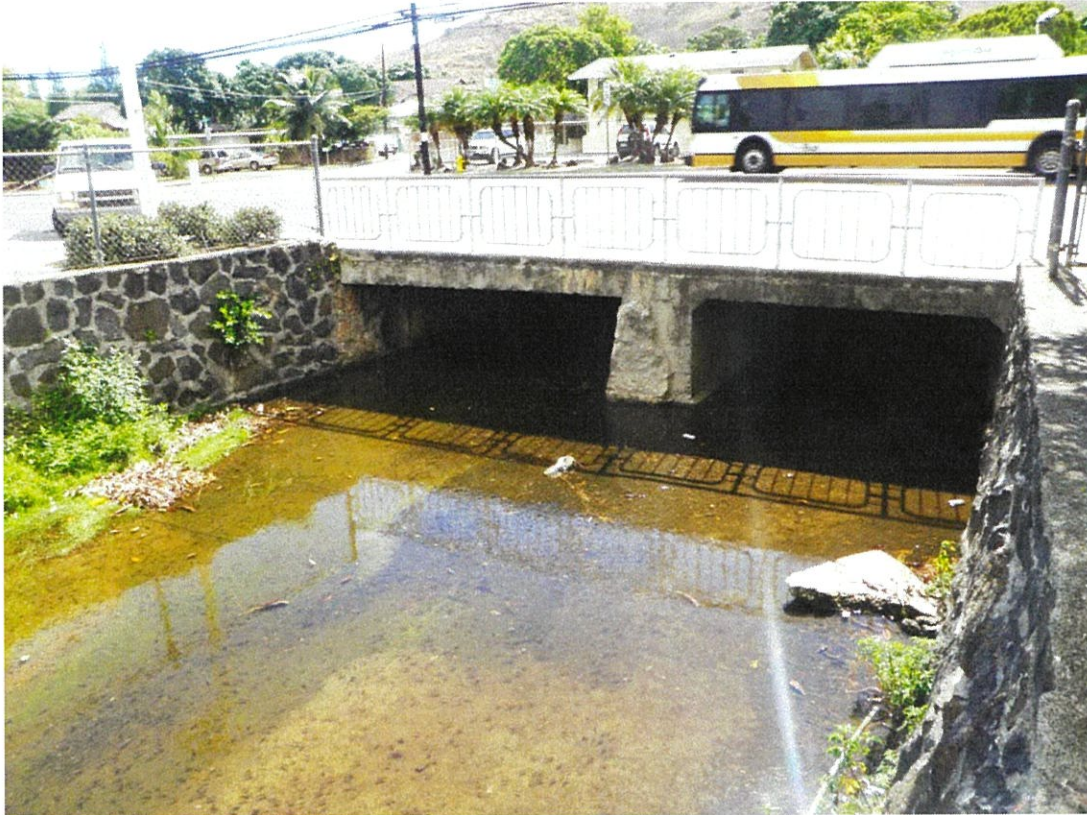
Photo 2-1 – Downstream of the Keolu Street Hele Channel culverts; proposed BMP location.
