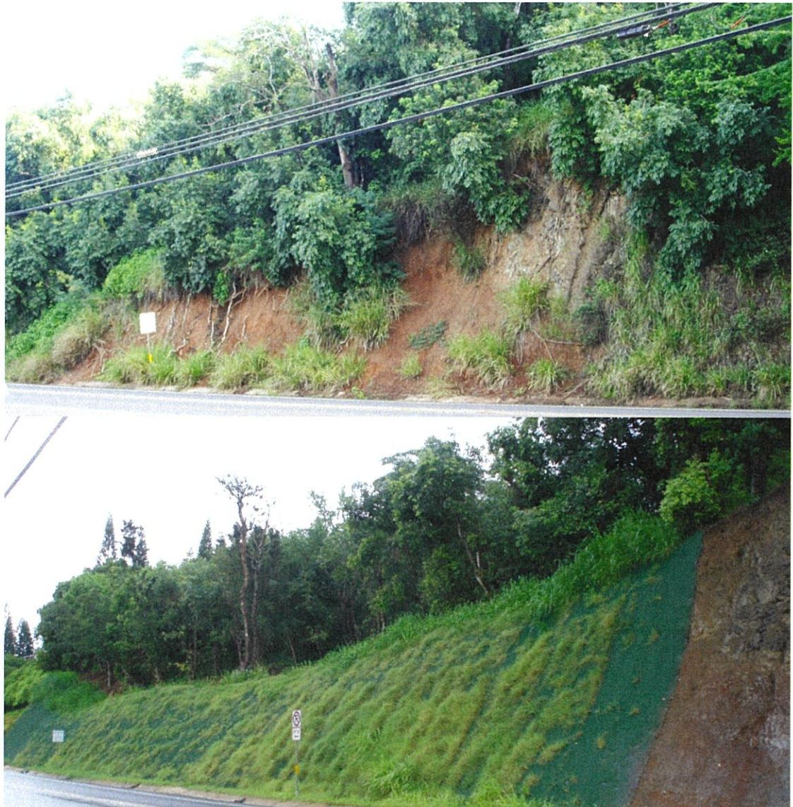
Photo 4 – Before and after photos of an anchored reinforced vegetation system.
