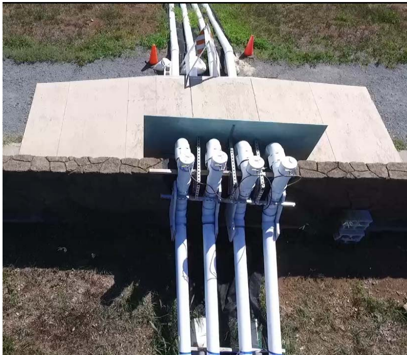
Figure 2.4. Syphon and pedestrian ramp across the levee.
