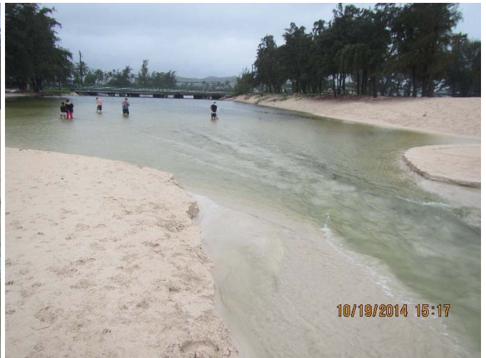
Figure 3.10 October 2014 the City responded to a high water surface in the pond and an impending rainstorm by conducting an “emergency” opening of the stream mouth. Flow established in a 1/2-foot deep 20 foot wide channel completed at 16:15. Flow and erosion first concentrate at the center of the channel and then widen into a 40-foot wide 3 foot deep channel in about an hour and fifteen minutes.
