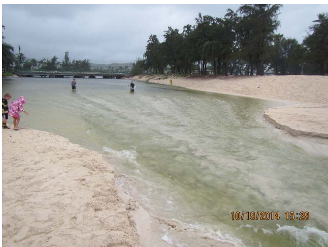
Figure 3.10 October 2014 the City responded to a high water surface in the pond and an impending rainstorm by conducting an “emergency” opening of the stream mouth. Flow established in a 1/2-foot deep 20 foot wide channel completed at 16:15. Flow and erosion first concentrate at the center of the channel and then widen into a 40-foot wide 3 foot deep channel in about an hour and fifteen minutes.
