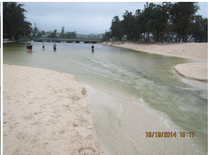
Figure 34. October 2014 the City responded to a high water surface in the pond and an impending rainstorm to conduct an “emergency” opening of the stream mouth. Flow established in a 1-foot deep 15 foot wide channel completed at 16:15 developed into a 30-foot wide 3 foot deep channel in about an hour and fifteen minutes. Within minutes of the last photo the cameraman had to abandon his location as the bank was eroding from beneath his feet.
