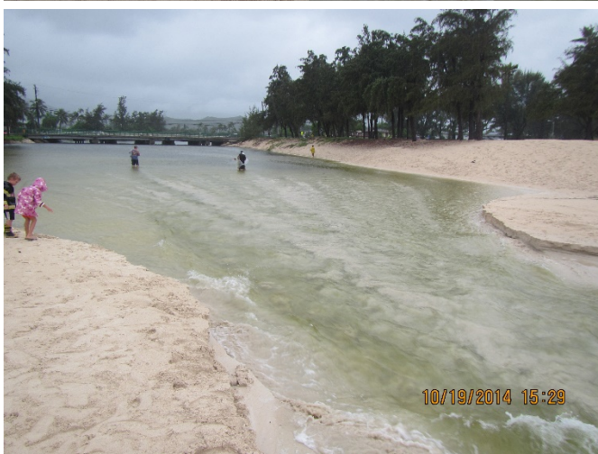
Figure 34. October 2014 the City responded to a high water surface in the pond and an impending rainstorm to conduct an “emergency” opening of the stream mouth. Flow established in a 1-foot deep 15 foot wide channel completed at 16:15 developed into a 30-foot wide 3 foot deep channel in about an hour and fifteen minutes. Within minutes of the last photo the cameraman had to abandon his location as the bank was eroding from beneath his feet.
