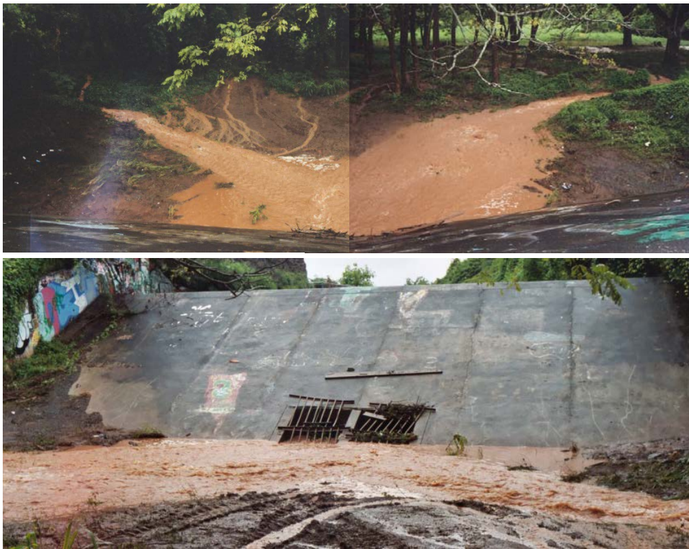
Figure 26. Top: Looking down the inside Keopu dam face as muddy water pours through the two erosional channels cut through the internal raised berm. Bottom: Inside the basin looking at the back of the dam face with the muddy water flowing into the two flow control structures beneath the dam.
