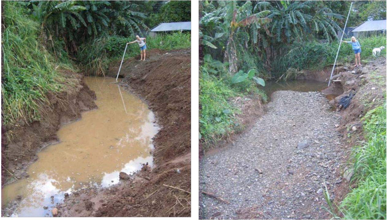
Figure 25. Before (left) and after(right) sediment from a City storm drain filled this swale during a single storm. The staff is a 16-foot survey rod.
