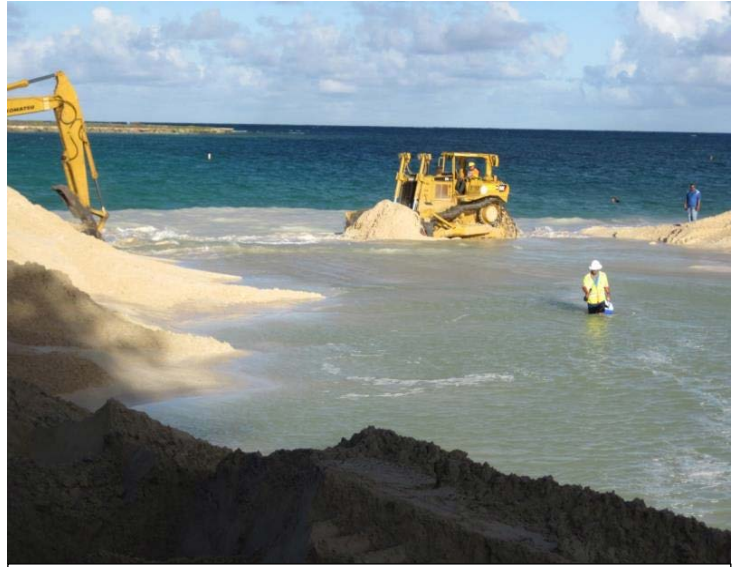
Figure 29 The City uses heavy equipment to open the stream mouth about nine times per year.
